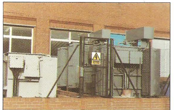
(Above) The 6MVA supply transformers.
